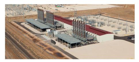
Antelope Station, near Abernathy, Texas, reached commercial operation on June 24, 2011. The plant can generate 165.4 MWs of natural gas-fired electricity. The plant consists of eighteen 9.34 MW Wartsilä reciprocating engine generators, each of which can achieve full output in five minutes.
