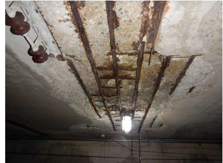
HRBT Invert Slab Concrete Repairs
