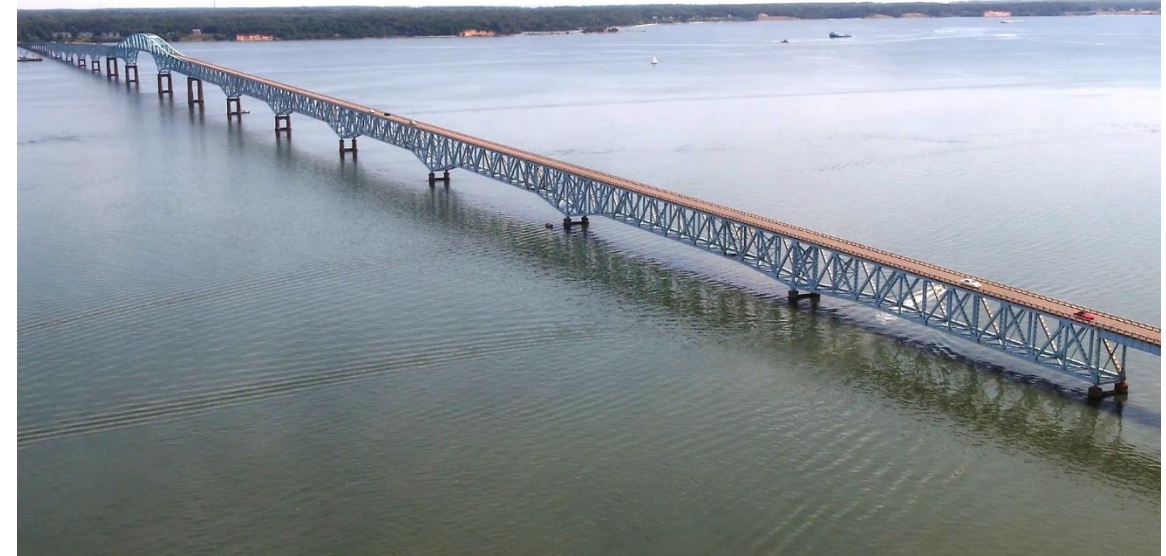
The Robert O. Norris Bridge carries Route 3 traffic over the Rappahannock River between Lancaster and Middlesex counties, linking the Northern Neck and Middle Peninsula
