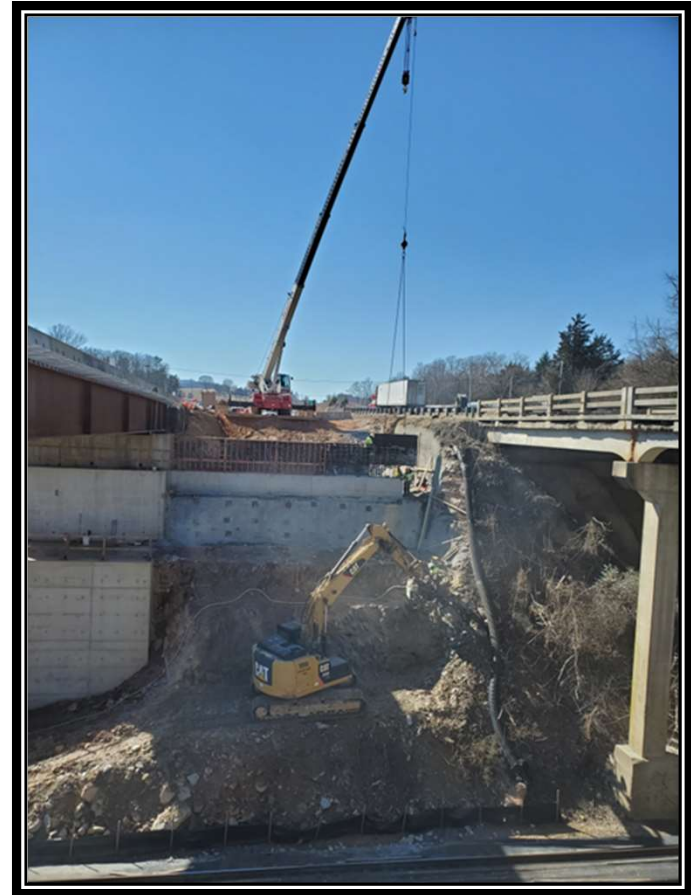
Installing soil nails with excavator
