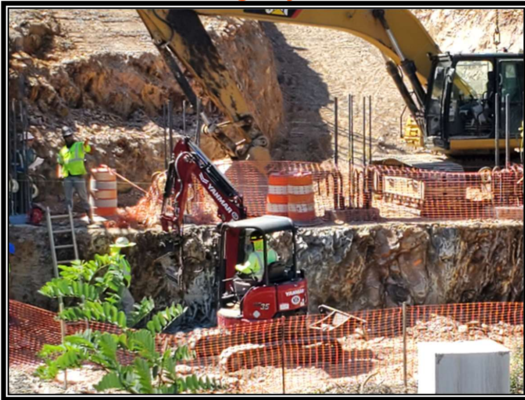
Mini Excavator with hoe ram set on ledge by crane
