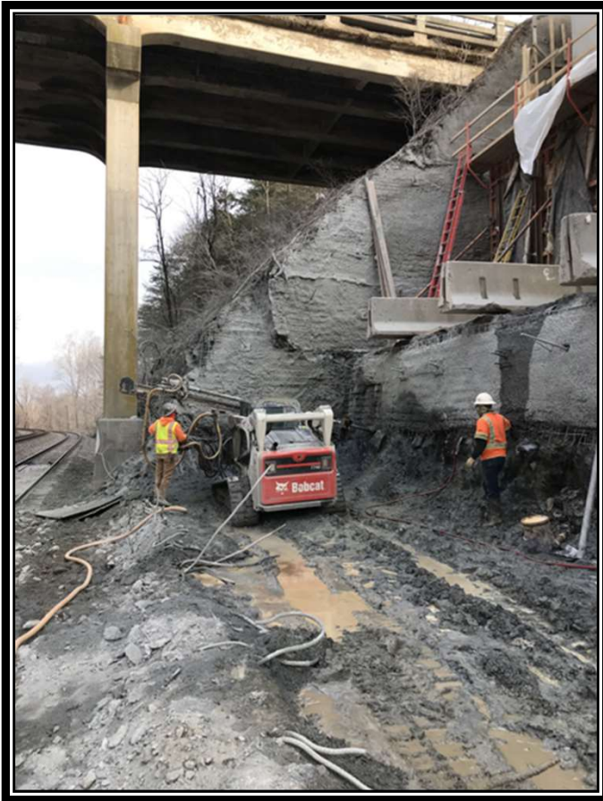
Installing soil nails with Bobcat
