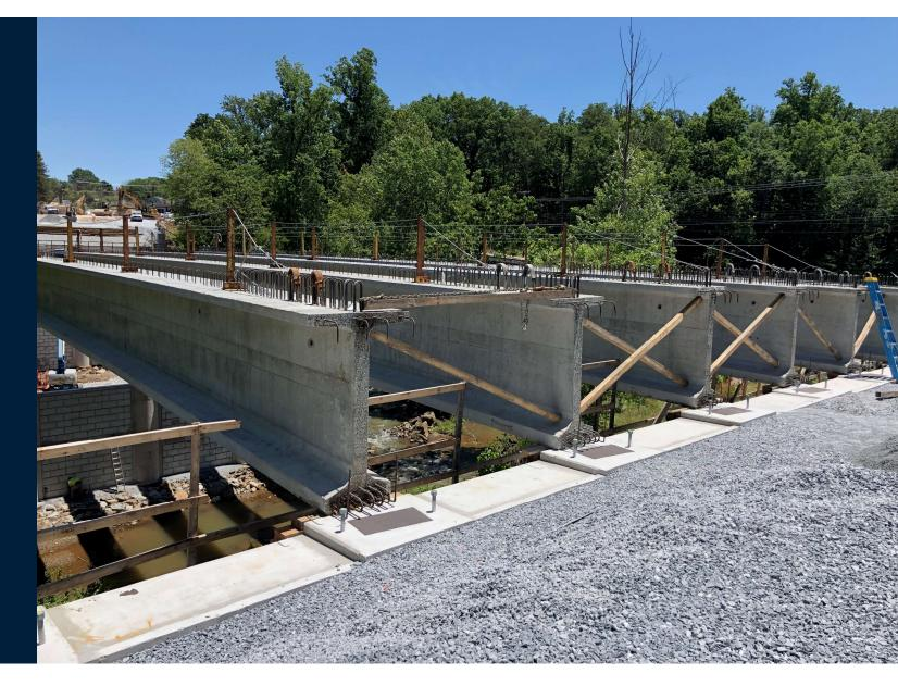
Semi-integral abutments on each end of the bridge
