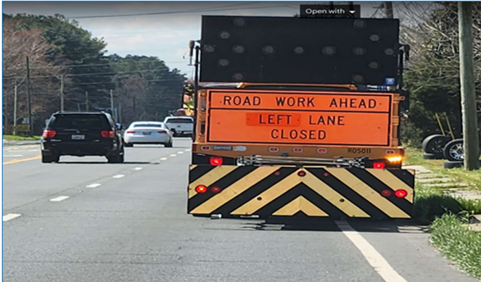
Incorrect work zone signage
