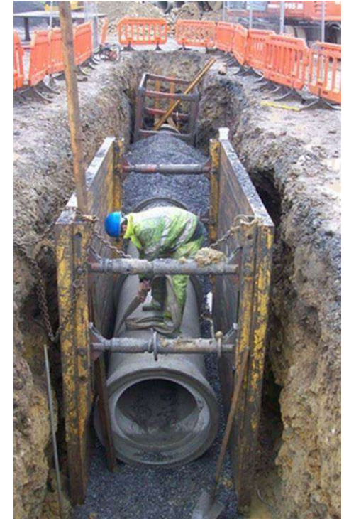
Example: Difficult, Low Production, High Unit Cost, Pipe Installation
