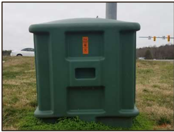
Telecommunications Pedestals
