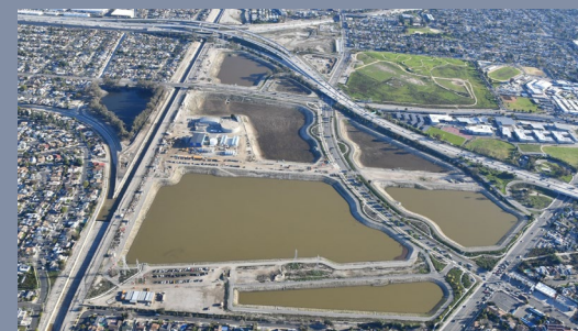
Tujunga Spreading Grounds Enhancement
