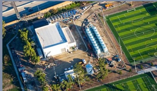
North Hollywood West Wellhead Treatment
