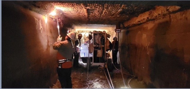
Los Angeles Aqueduct Old Top Removal
