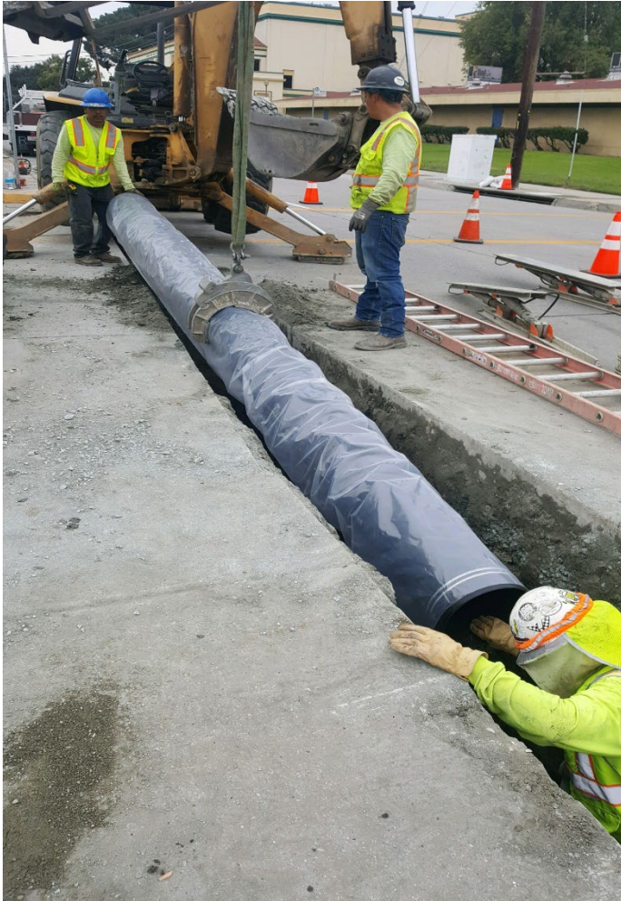
CIP# 7440 12-inch Watermain Installation
