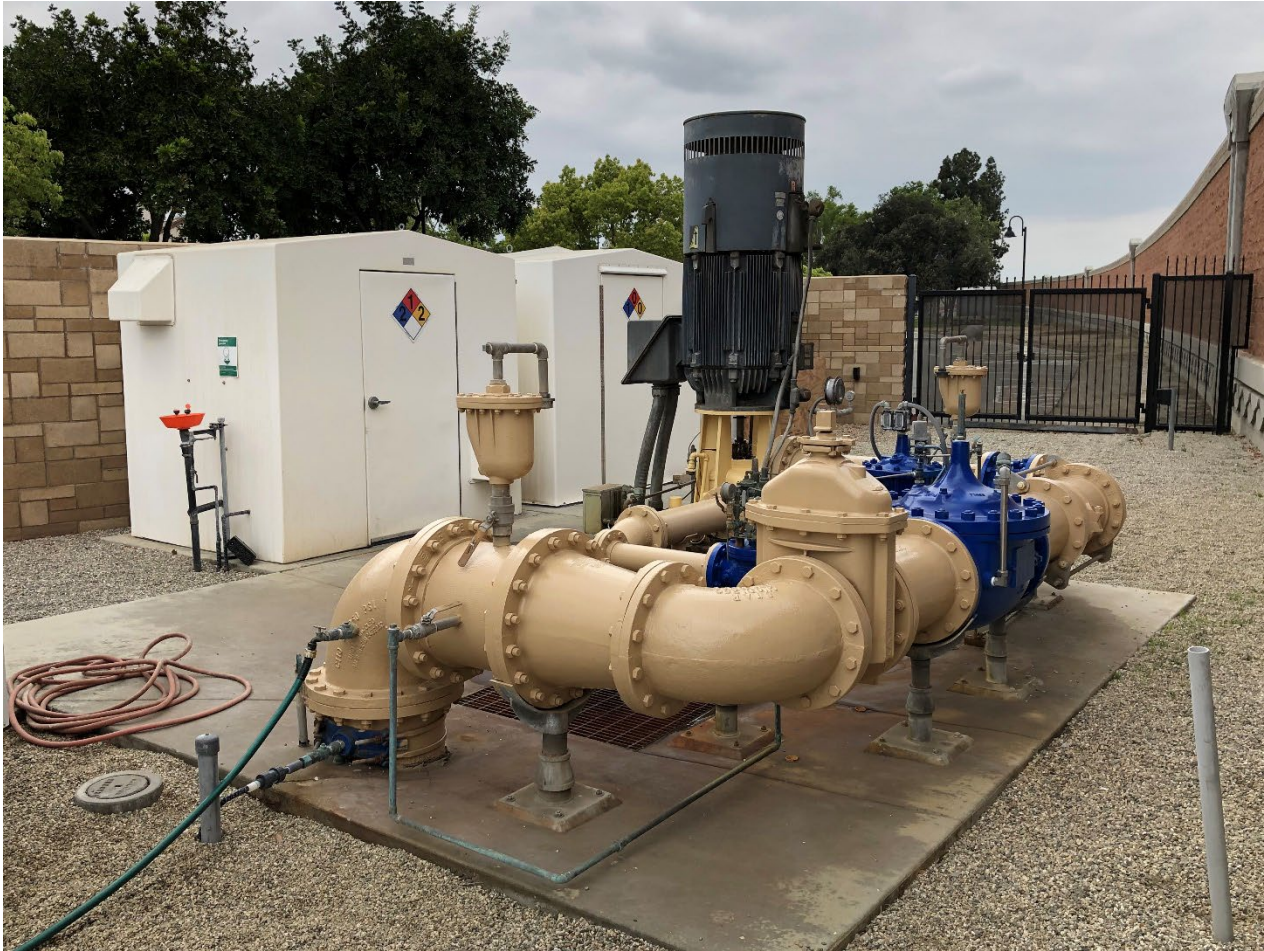
Well 10 Control Valve Upgrades
