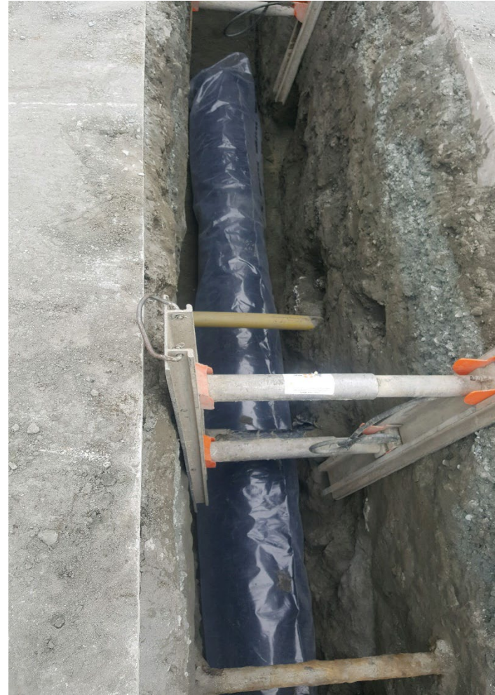
CIP# 7440 12-inch Watermain Installation
