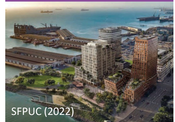
Mission Rock at Third and Mission Rock Street – San Francisco, CA
