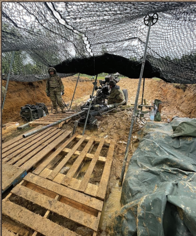
5th Section's defilade position with adequate depth, width, and length. The position was constructed with the berm to the rear and ramp forward. Constant precipitation with the clay soil led to the section constructing flooring using ammo pallets and ammo boxes to gain traction.
