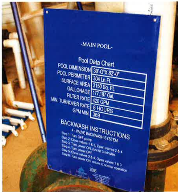
Photo 15-5. Having the pool parameters and instructions on how to backwash the pool helps minimize mistakes.
