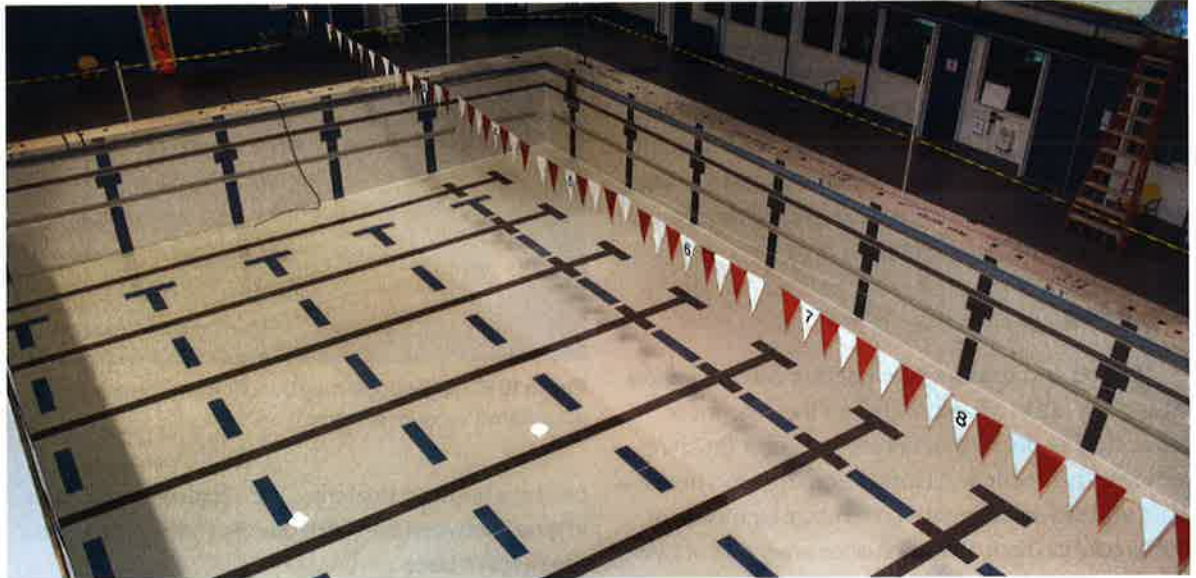
Photo 16-6. Care must be taken not to damage the glaze on tiles. Always use a non-abrasive cleaner.
