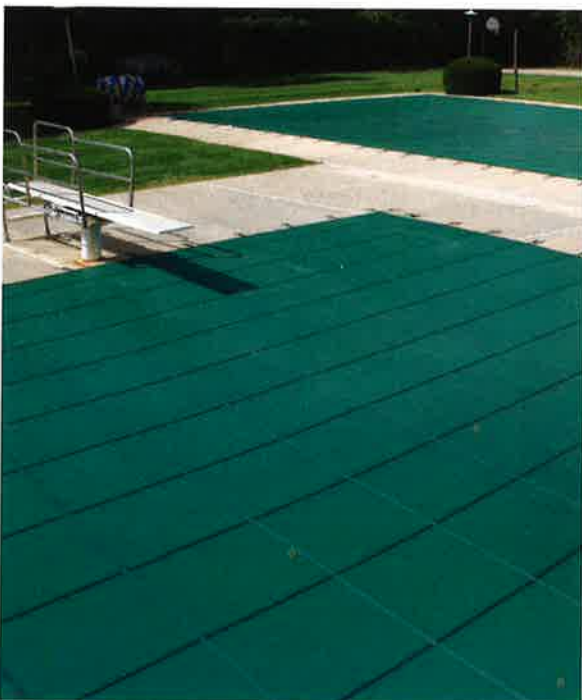
Photo 16-9. Most winter covers are fastened to the decks around the pool by a spring-loaded device.
