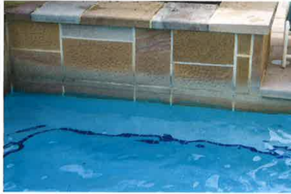
Photo 7-8. Once the scum line starts to form, it may grow by attracting more contaminants from the water.
