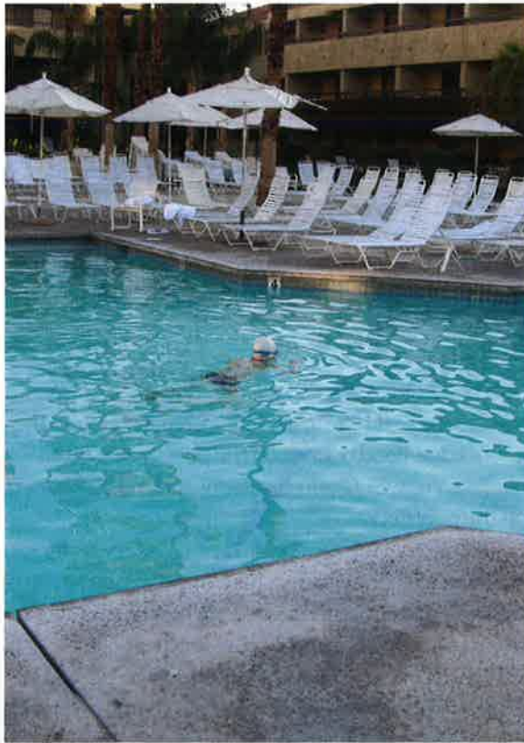
Photo 14-20. There should be adequate clearance around the pool to avoid tripping near the water's edge.
