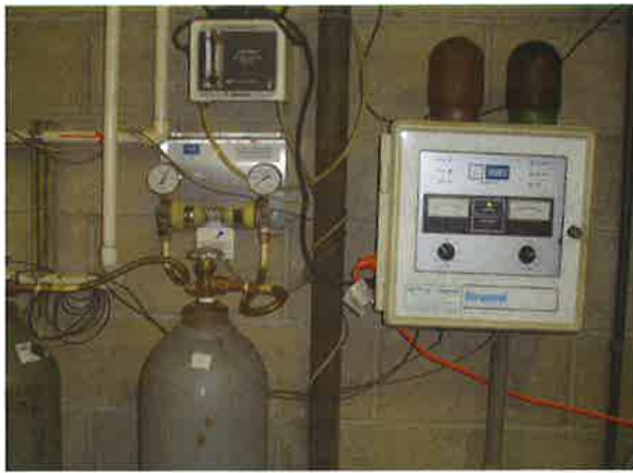
Photo 9-11. Carbon dioxide may be used instead of acids to lower the pH of pool/spa water.
