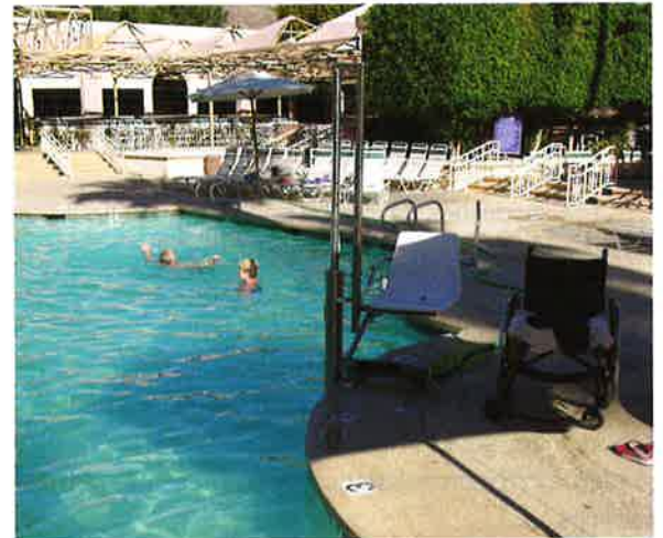
Photo 2-6. A pool lift may be a requirement for your facility.
