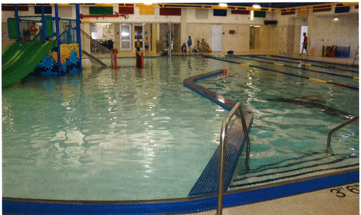
Photo 12-8. Humidity control is an important design consideration for large indoor pool facilities.
