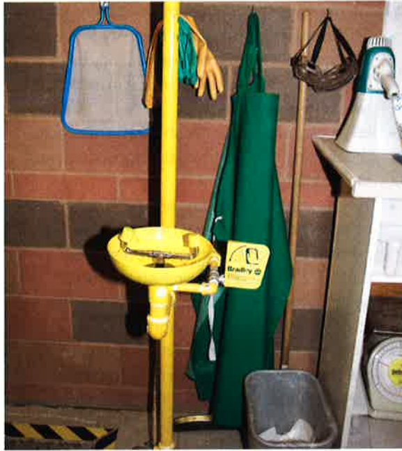
Photo 14-24. There should be ready access to eye and body wash stations for the removal of chemicals, as well as personal protective equipment.
