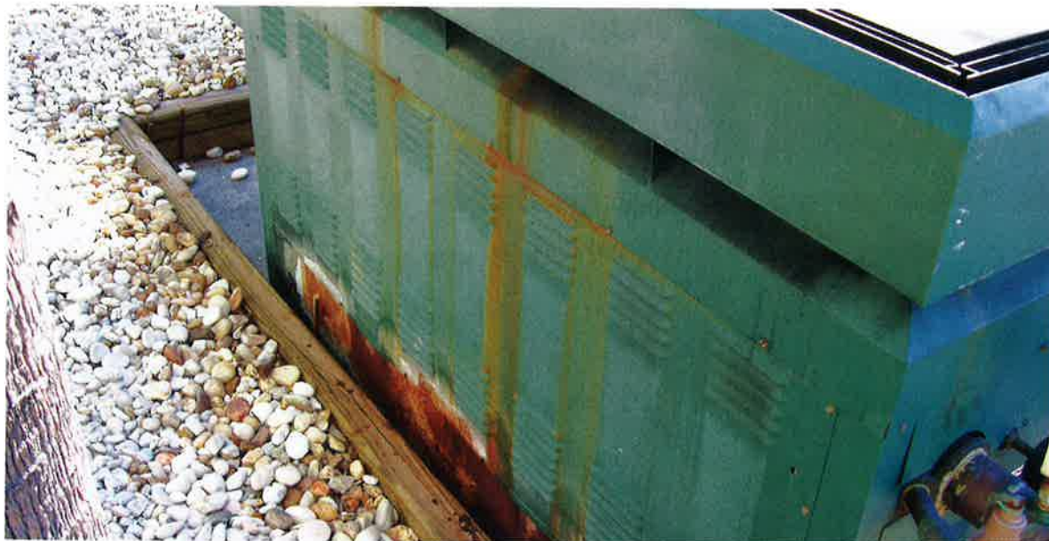
Photo 17-6. Gas-fired pool/spa heaters must be installed so as to not be affected by water run-off from roofs.
