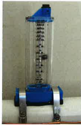
Photo 10-13. Flow meters are generally mounted on the return piping after all other system components but before any chemical feed injection.
