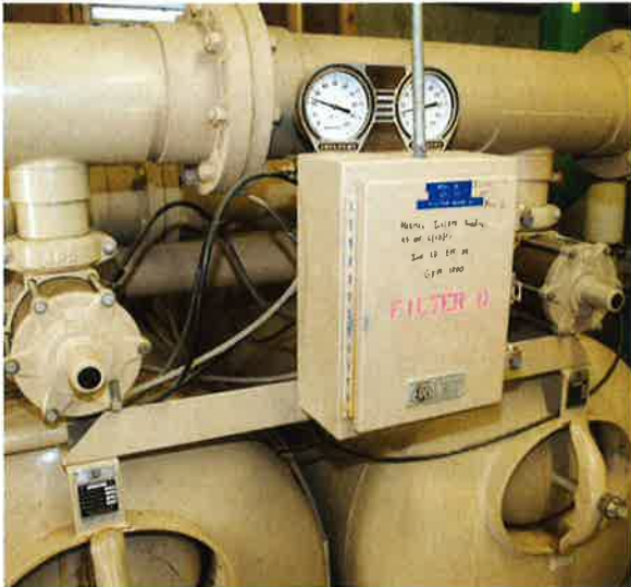
Photo 10-9. Butterfly valves with electric actuator
