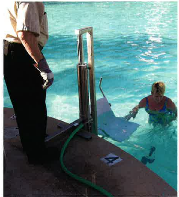
Photo 18-11. Pool lifts should be user-operated and not require the assistance of others.
