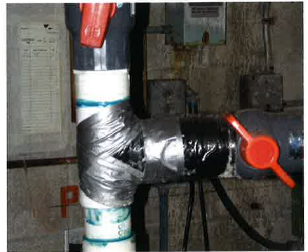
Photo 17-2. All repairs should be done in a professional manner to protect people and equipment.
