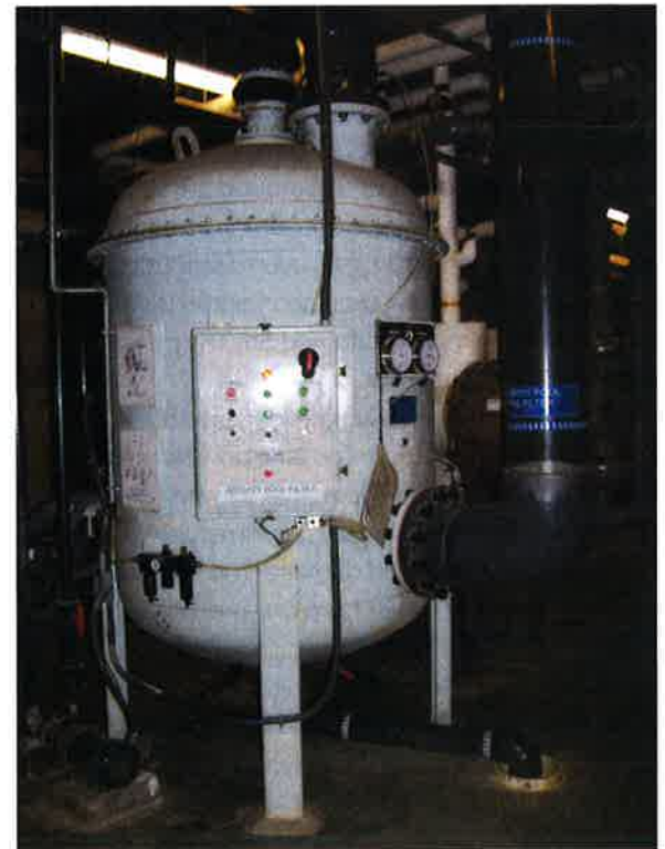
Photo 11-8. Regenerative filters require a much smaller footprint for installation compared to sand filters.
