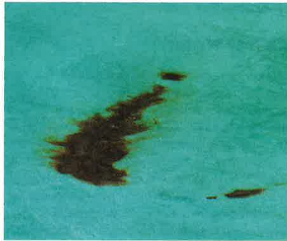
Photo 7-5. It is important that the source of stains be identified. Dark stains are often the result of plant matter that falls to the bottom of the pool.
