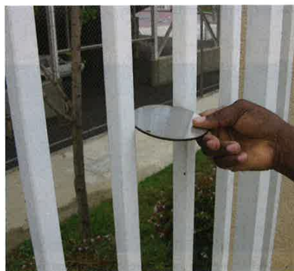
Photo 14-3. Openings in the barrier should not allow passage of a 4-inch (10 cm) diameter sphere or disk.
