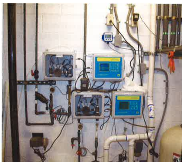
Photo 8-15. The ORP probe reading signals a controller to turn on or off chemical feeders.
