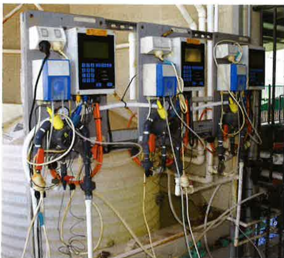
Photo 13-7. An ORP system for chemical control is often required by codes for spas, which helps to maintain proper disinfectant levels.
