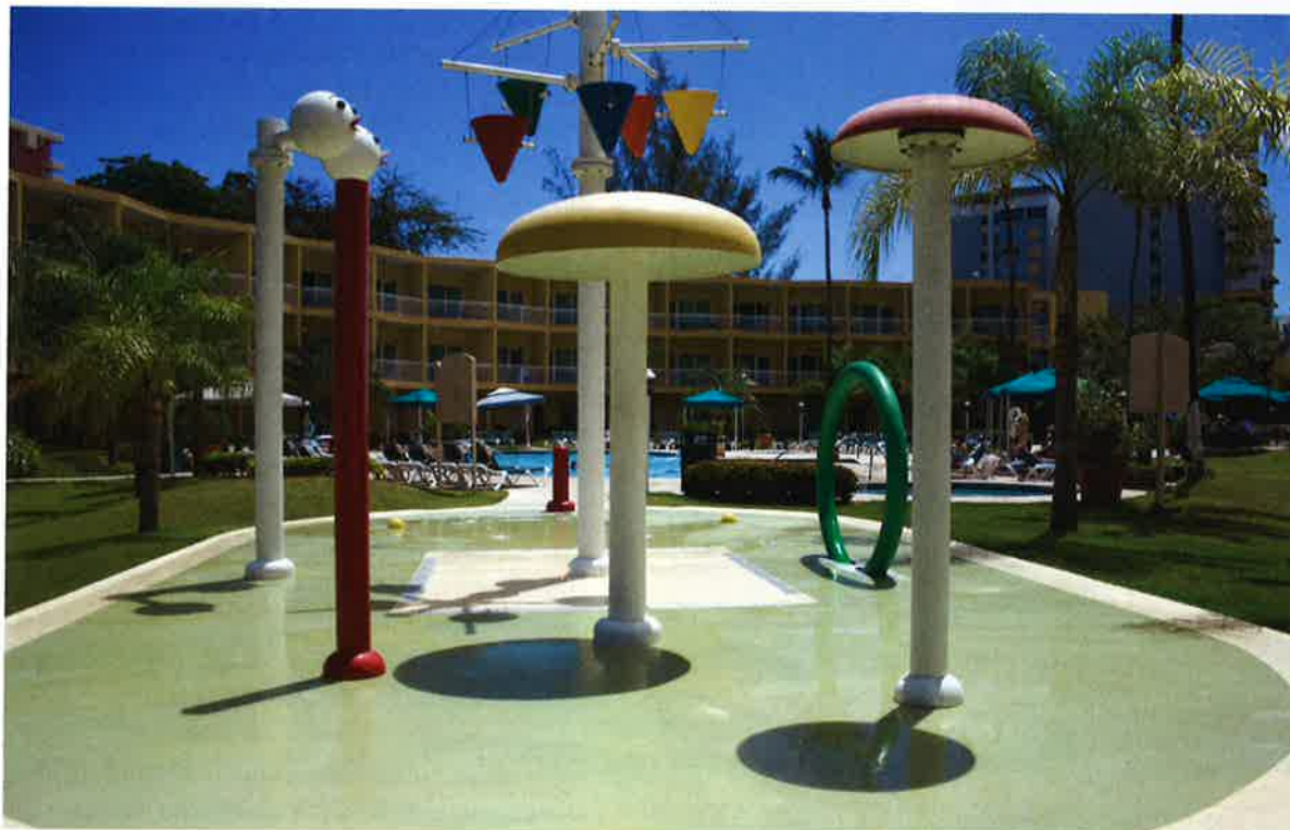
Photo 16-1. Maintenance systems can be simple or complex, depending on the design and use of the facility.
