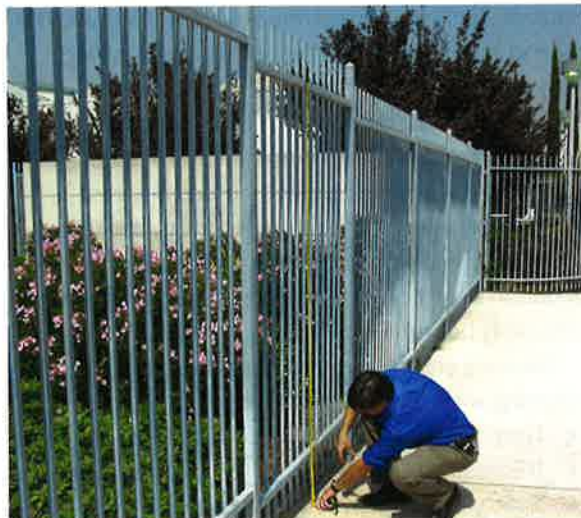
Photo 16-4. Inspection of the grounds must include barriers and gates.
