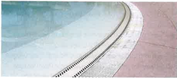
Photo 18-13. Zero depth or beach entry is an alternative way to allow people with disabilities to access the water, even in a wheelchair.
