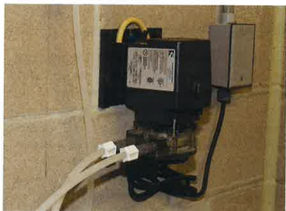
Photo 9-1. The operator should check the face plate on the feeder to verify that it has been tested and certified by a recognized organization.
