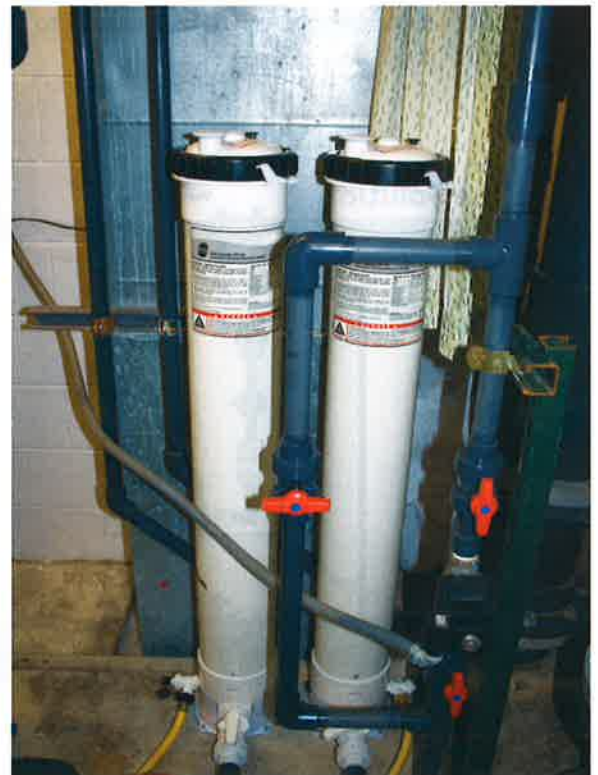
Photo 9-6. Erosion feeders use a stream of water to contact the dry chemical, causing the chemical to erode and dissolve.
