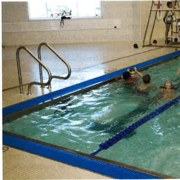
Photo 10-3. A rim-flow gutter system with grating. Since users come in direct contact with the grating in a rim-flow system, the grating should have tamper proof fasteners holding it in place.
