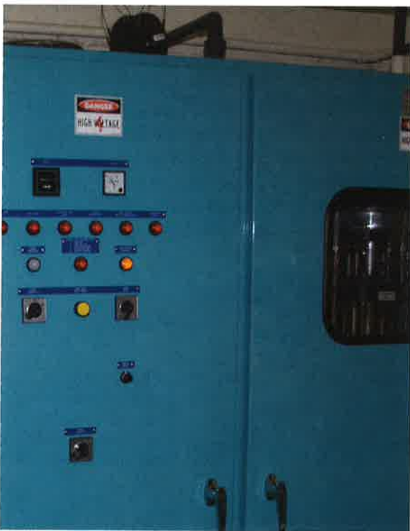
Photo 9-12. A corona discharge ozone generator may have a contact column to increase the mixing time to achieve the greatest amount of ozone in solution.
