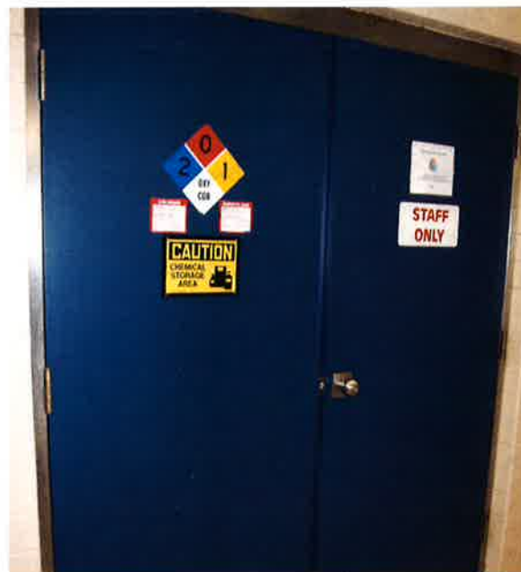
Photo 14-17. Signs should warn of chemical hazards related to storage.
