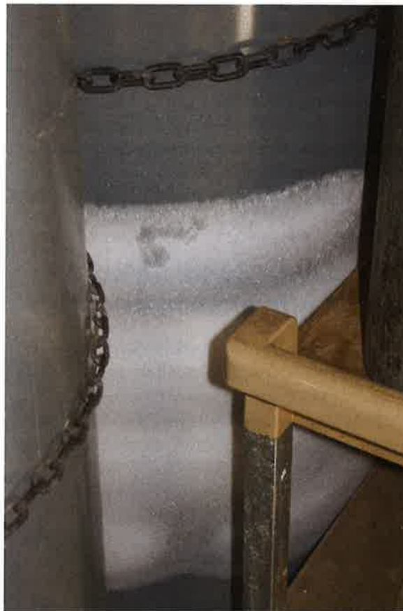
Photo 2-2. Gas chlorine use requires proper training concerning handling and storage. Cylinders must be individually chained to the wall and the regulator flow must be slow enough to prevent ice formation on the cylinder.
