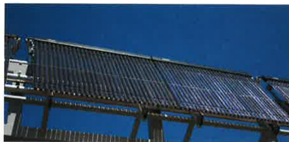
Photo 12-6. Solar panels absorb heat energy from the sun, which is then transferred to the water.
