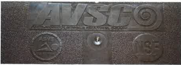
Photo 2-7. Pool circulation equipment should bear the proper regulatory certification markings.
