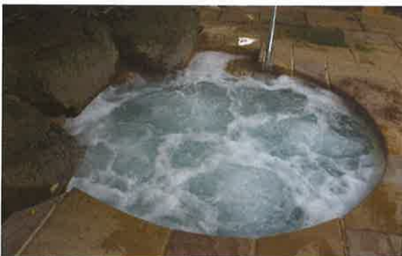
Photo 7-7. The aeration from the therapy jets can increase the foaming in a spa.
