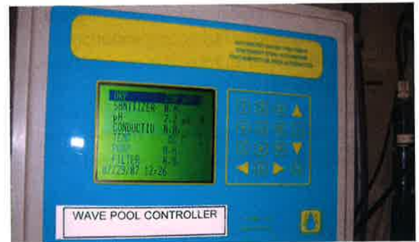
Photo 9-18. Some ORP control systems will display pH and ORP levels and have warning alarms.
