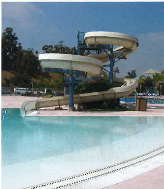
Photo 3-3. Evaporation, splash out, and leaks contribute to water loss that must be replaced.
