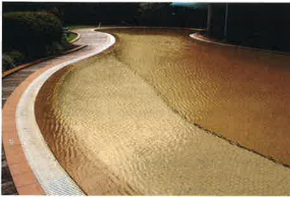
Photo 7-4. Iron in the source water can give a reddish-brown color to the water in the pool.
