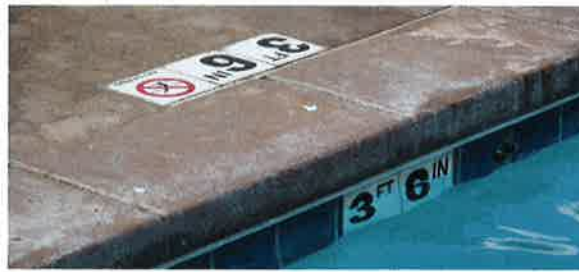
Photo 14-19. Many codes require depth marking signs. It may be advisable to have the markings in both feet and meters.
