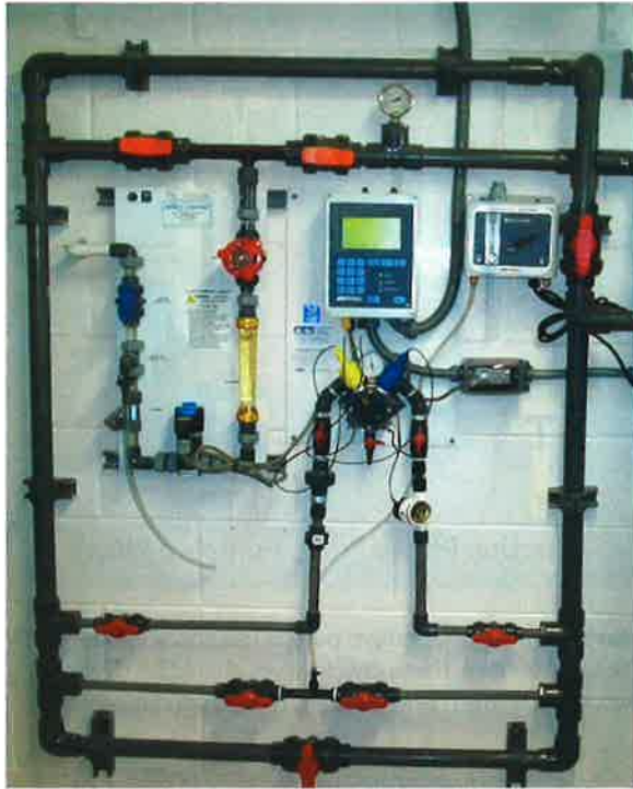
Photo 9-5. Chemicals can be evenly distributed throughout the pool system through liquid solution feeders.
