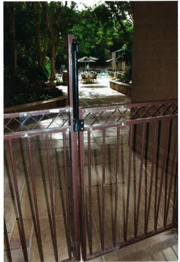
Photo 18-7. Suitable barriers should be designed to prevent unauthorized access.
