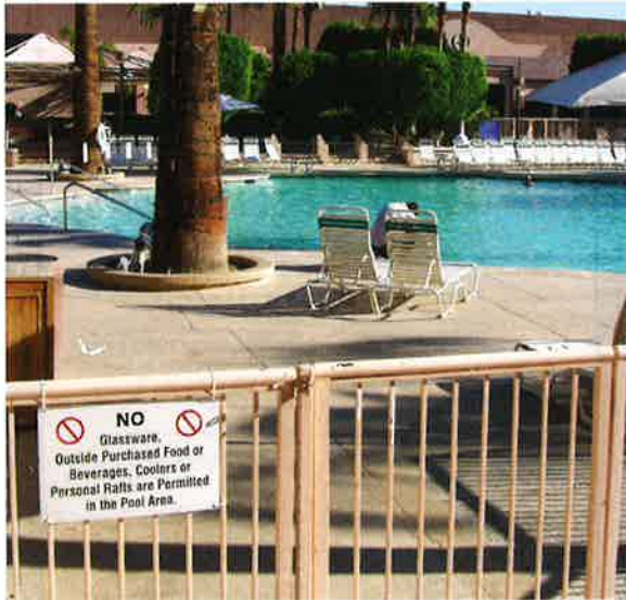
Photo 2-5. A small child can open this gate. The CPSC provides guidelines covering gates and latches for proper installation.
