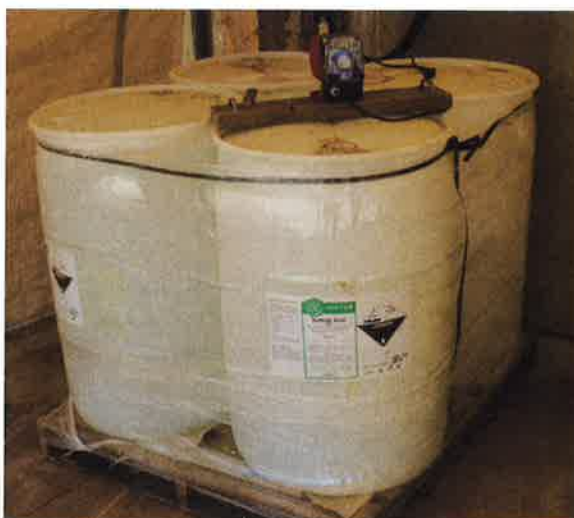
Photo 14-22. Chemicals must be stored so that the container and packaging are not damaged by contact with water, even if they are packaged in drums.
