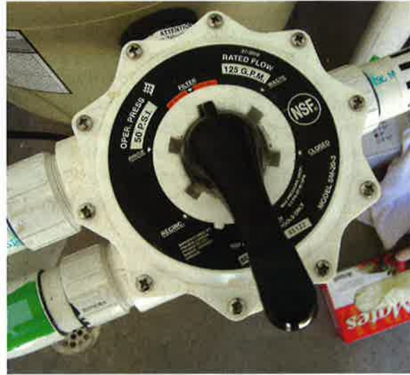
Photo 10-10. Some rotary valves have bypass, rinse, circulate, and on-off positions.
