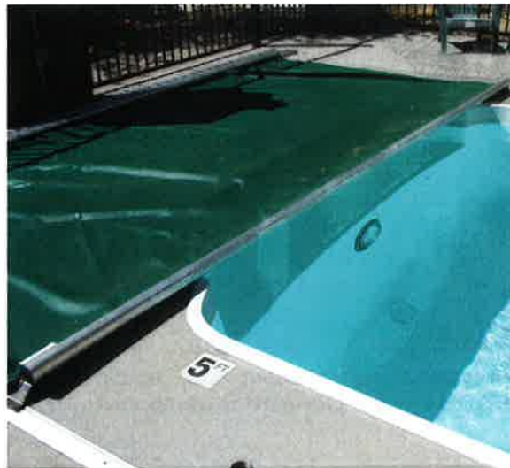
Photo 12-3. Fully automatic pool cover with a motor reel system that pulls the cover into place
