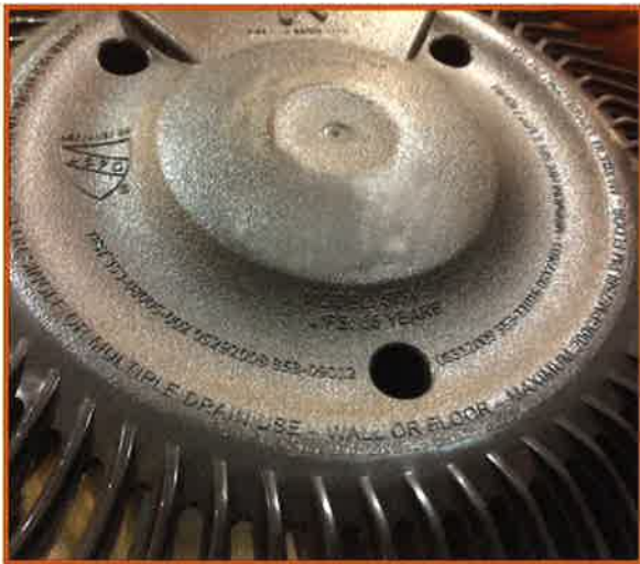
Photo C1-4: Example of compliant drain cover markings
