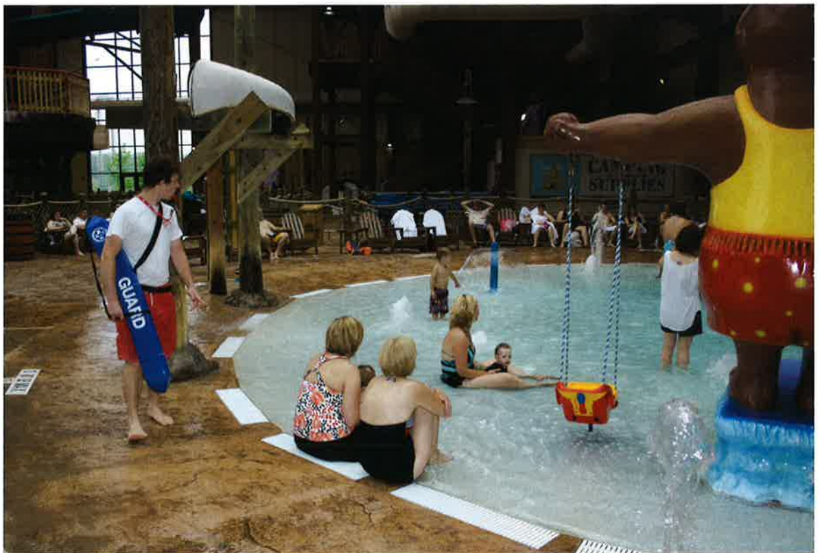
Photo C2-2. Each wading pool must provide at least one sloped entry into the deepest part.
