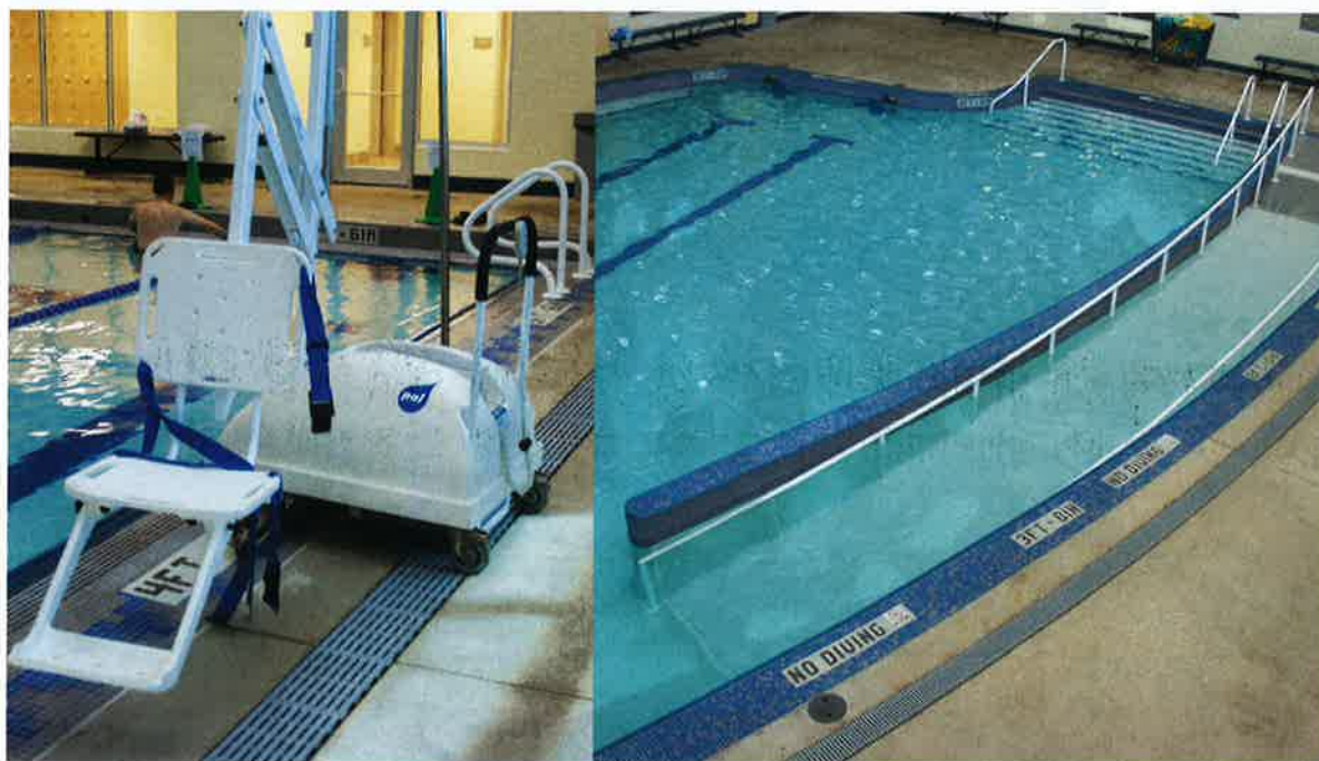
Photo C2-1: A swimming pool with two accessible points of entry.
