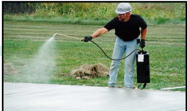
Spray-on curing compound
