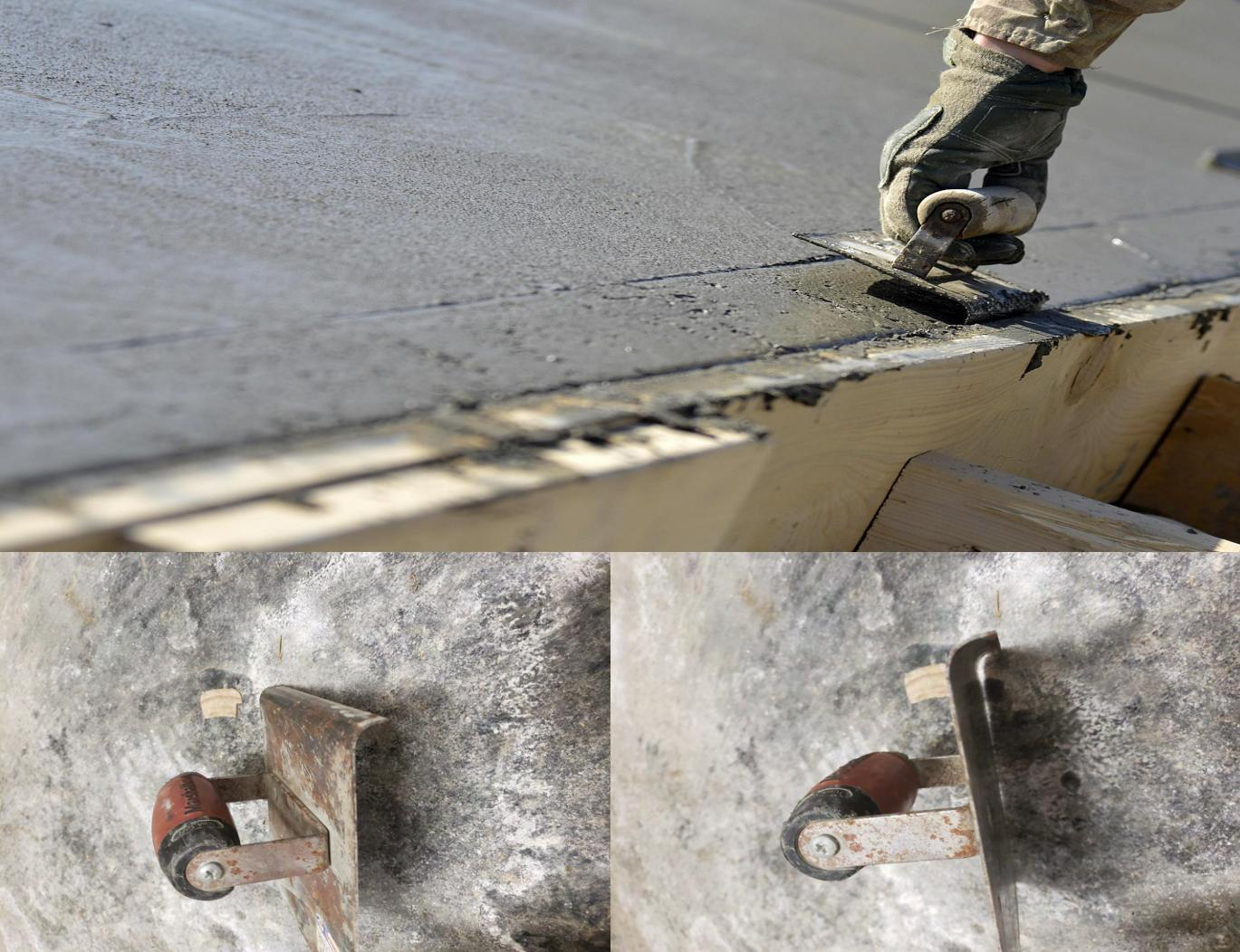
Edgers are used to create a better looking, more durable edge for a slab. Edging is often done several times throughout the finishing process. See Page 65 for more information and see Figure 7.10 for a picture of a walking edger.
