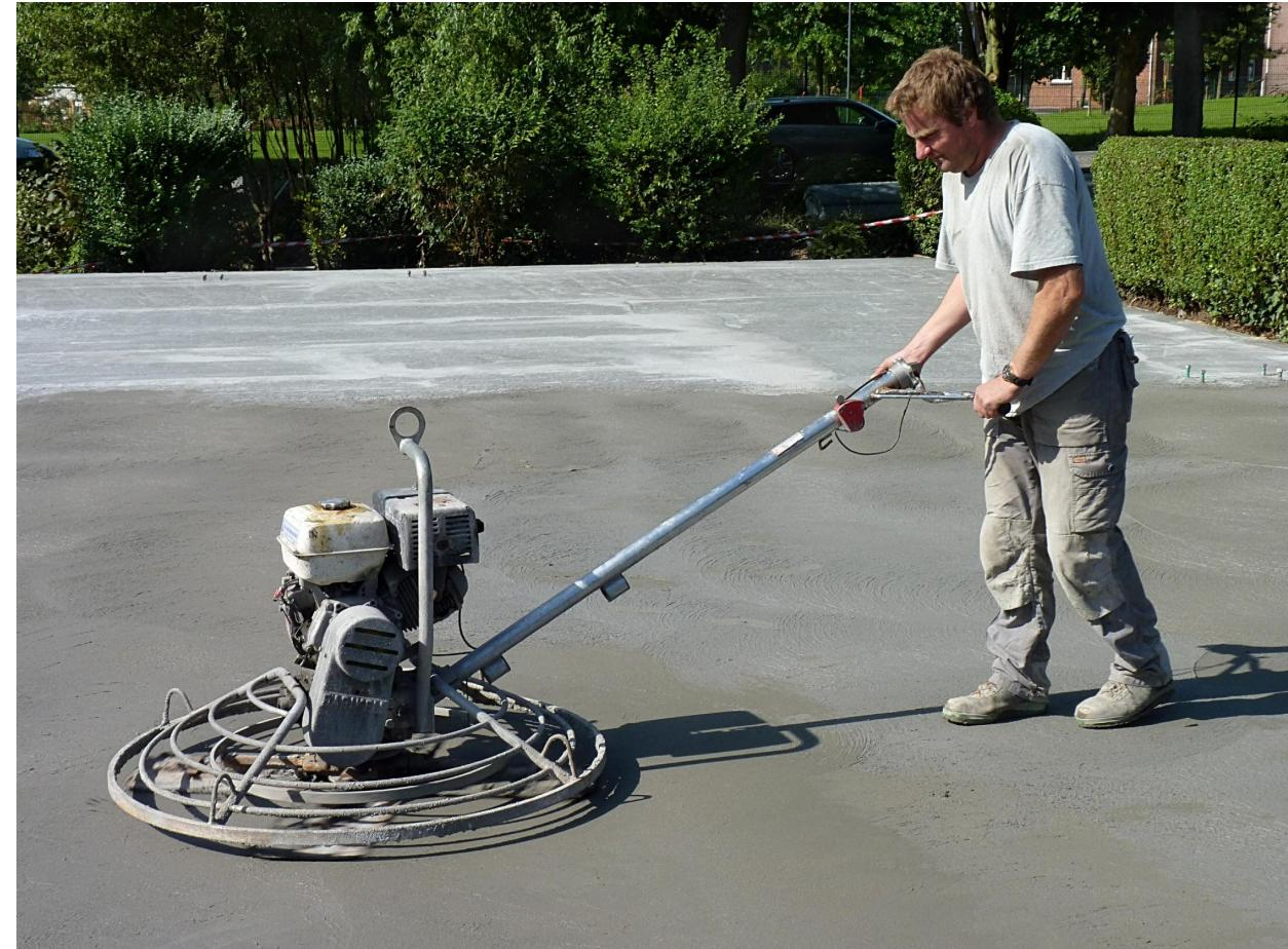
Walk-behind trowels are very common and are typically used for both floating and troweling concrete slabs. Always used after bleed water has gone and the slab has stiffened, the blades will be held nearly flat for floating and then gradually tilted up to begin troweling as the concrete continues to harden. See Pages 66-70 for important information.
