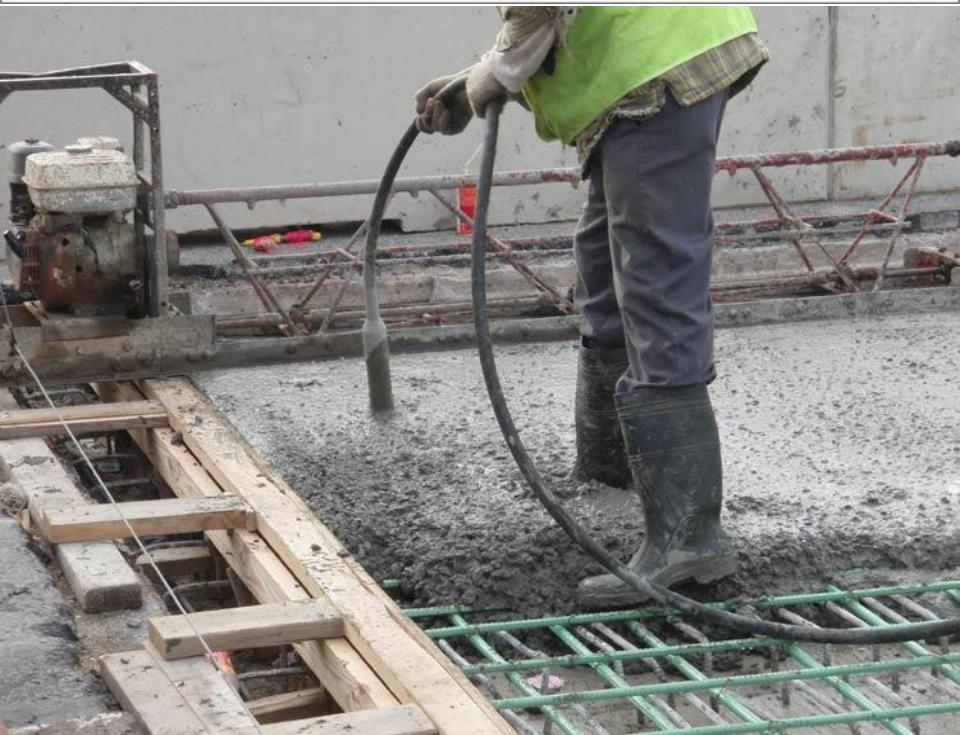
Not all slabs require internal vibration but slabs with lots of reinforcing (like the one in the picture) and thicker slabs (over 6 inches thick) may need to be consolidated with a vibrator like the one shown here. More information on types of vibrators can be found on Page 52 of the textbook.
