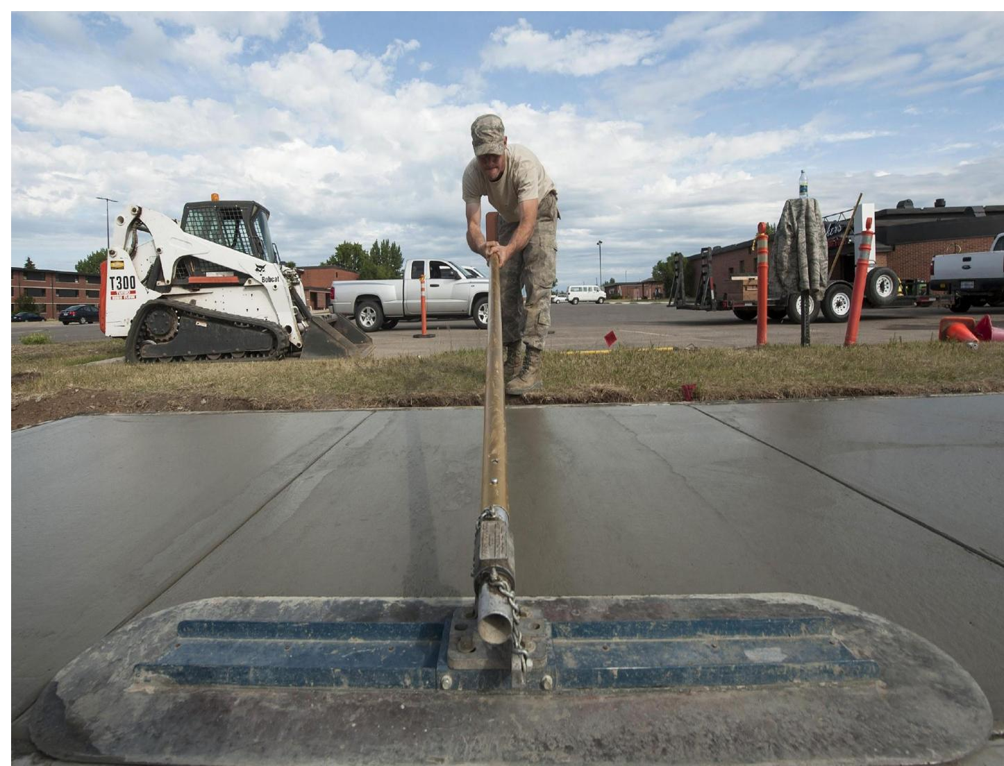
A **fresno** is a steel trowel and should **NEVER** be used until after all bleed water has disappeared and the slab is ready for a steel trowel tool.
