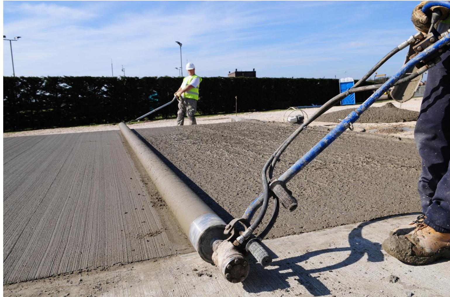
**Roller-screeds can be used for many types of slabs, including pervious concrete.**
