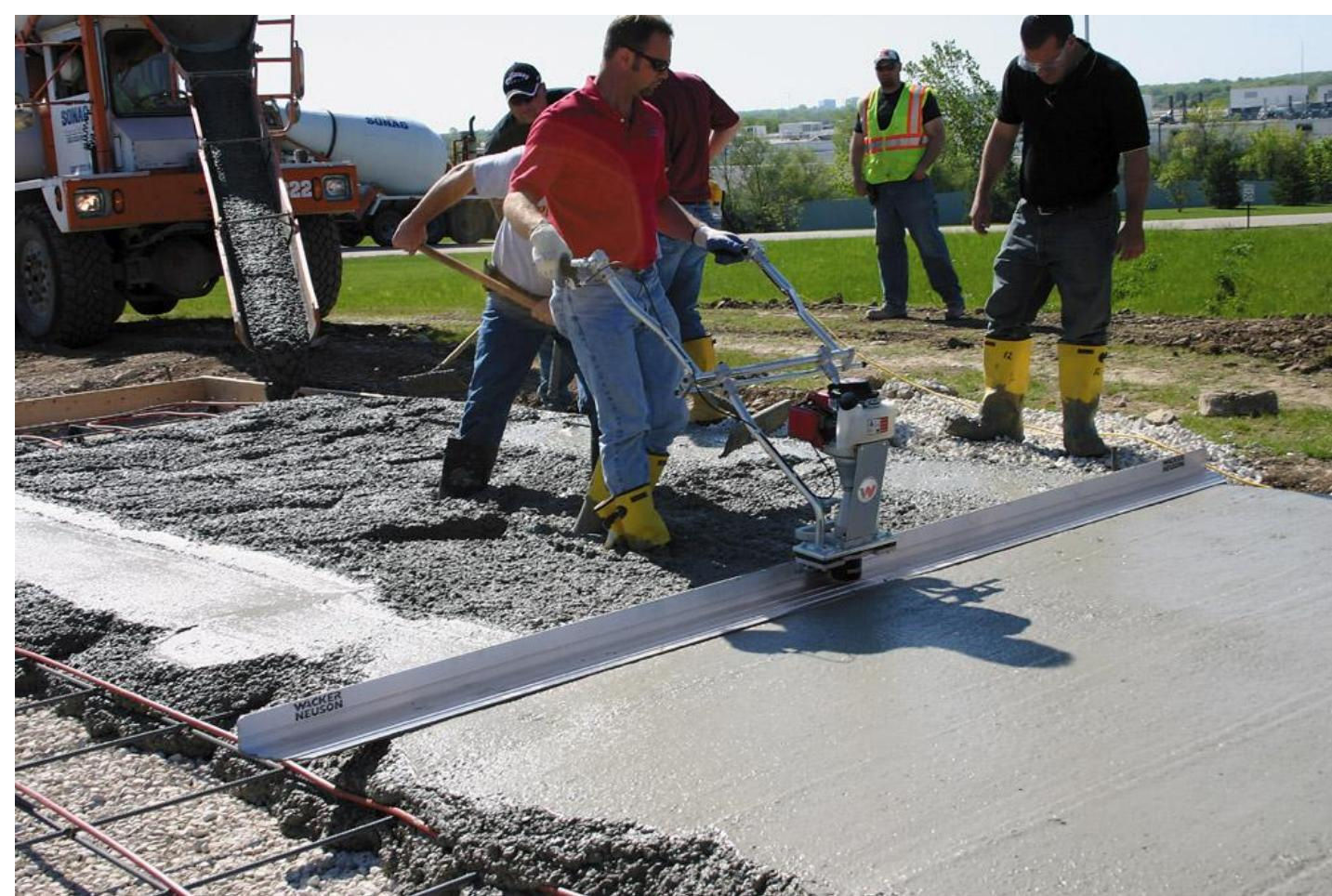
Hand-held vibrating screeds are often used on slabs without strict flatness requirements and in conjunction with “wet screeds” as shown above. Wet Screeds are strips of concrete that have been floated to the required elevation. See page 62 for more information.
