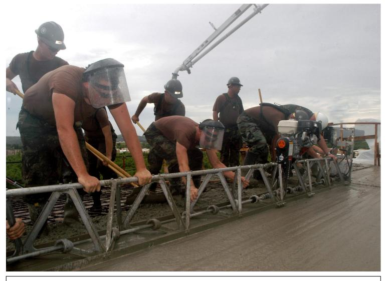
Often used for wide slab placements. These screeds typically vibrate as they strike-off the concrete surface.
