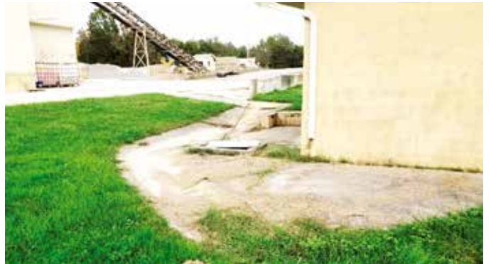
Storm Water Drainage Channel
