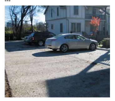
n July 27, 2015, a hot and humid day, around high noon— 54 yards of pervious driveway were placed to mitigate storm water run-off. Pervious concrete was selected because of its added benefits of filtering storm water pollutants and replenishing the aquifers below the surface. The surrounding sidewalks that lead into the townhomes' courtyard are also pervious concrete. The residential parking lot is located within the affluent Salemtown community, and the pervious concrete has added curb appeal.
