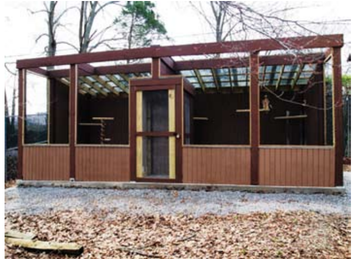
Figure 6. Nearly Completed Raptor Shelter
