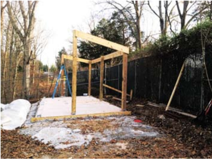
Figure 3. Frame Construction
