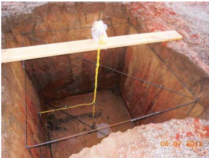
Figure 4: Excavation with Rebar Frame and Temperature Sensors
