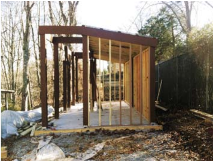
Figure 4. Further Frame Construction
