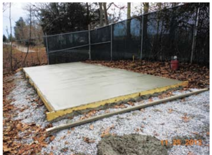
Figure 2. Finished Slab
