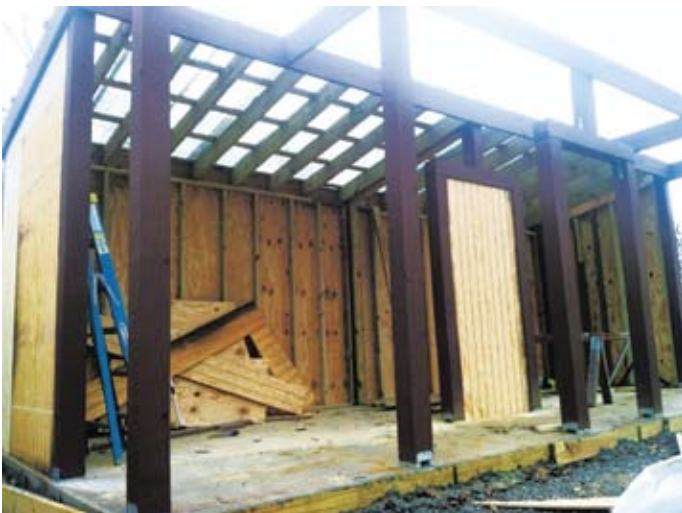
Figure 5. Sheathing Installation
