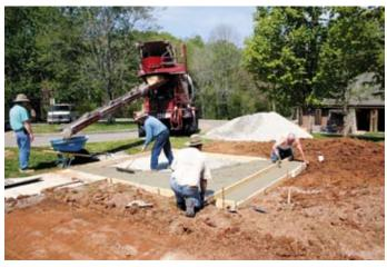
Figure 3: Close Up Showing Grading, Screeding and PCC Sampling
