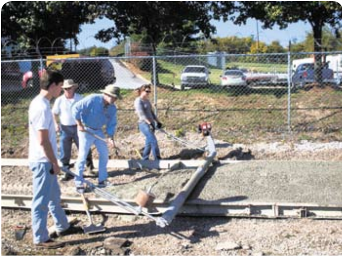
Figure 1: Light Compaction Typical for Pervious Concrete in Tennessee
