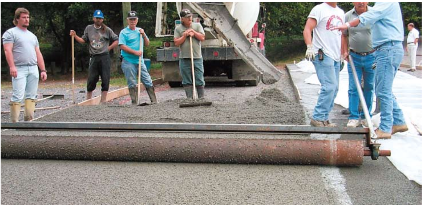
FIGURE 6. HEAVY HAND ROLLER COMPACTION AT KINGSPORT GREENWAY, 2001
