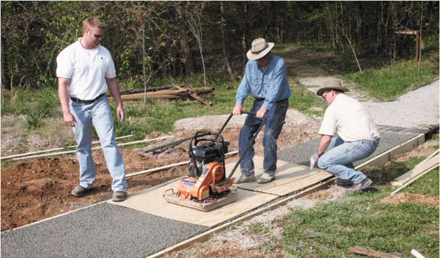
FIGURE 5. VIBRATORY PLATE COMPACTION AT BURGESS FALLS STATE PARK APRIL 19, 2005
