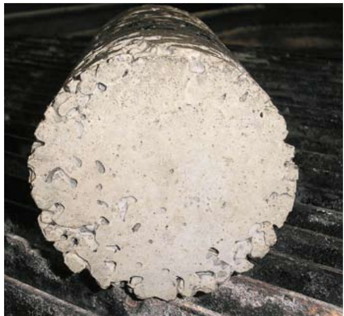
Figure 1. Severe Paste Drain Down
