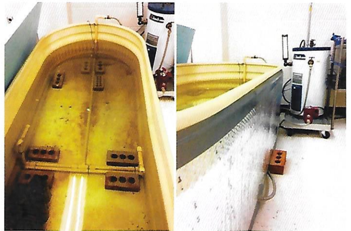
Figure 7: Plumbing for Accelerated Curing: Internal (left); External (right)
