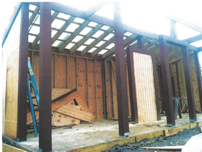
Figure 5. Sheathing Installation
