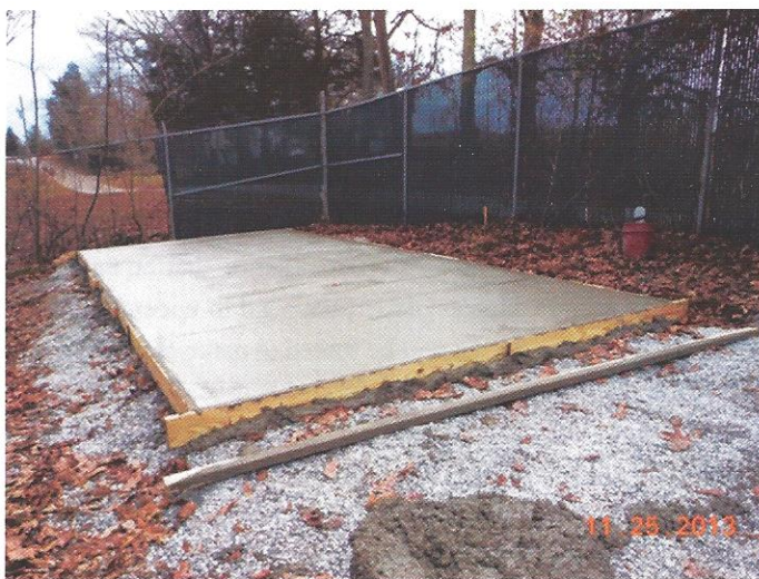
Figure 2. Finished Slab
