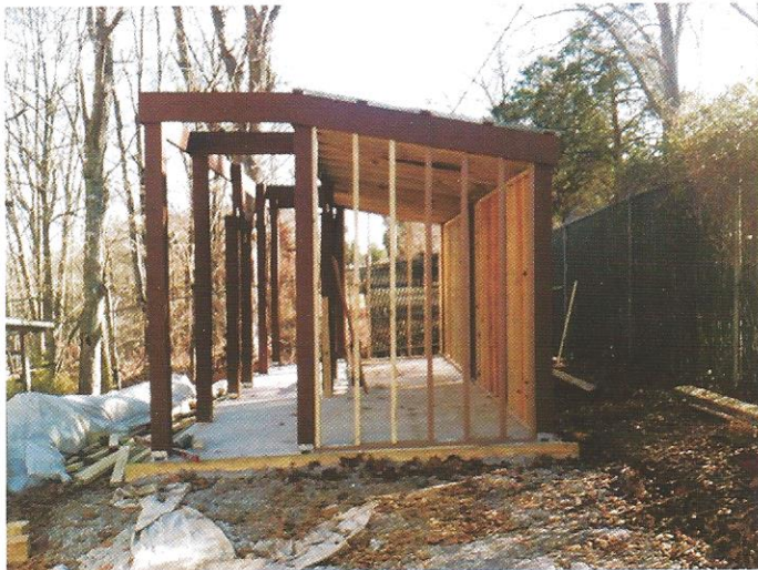
Figure 4. Further Frame Construction
