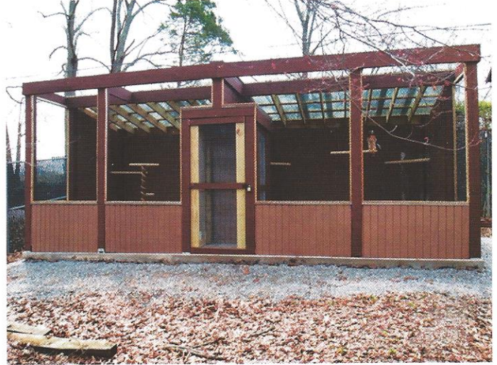
Figure 6. Nearly Completed Raptor Shelter
