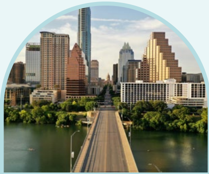
Bat Bridge Booster $2,500
