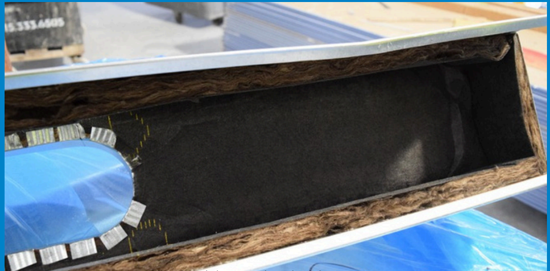
Insulated duct used on the job
