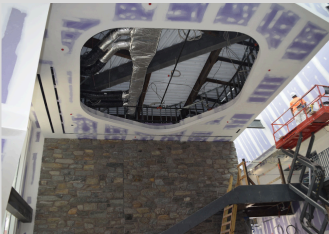
HVAC work inside the school's entrance
