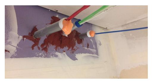
A non-firestop foam has been used inside the conduits
