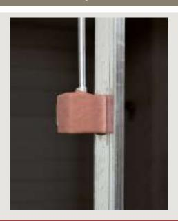
Firestop is used to seal openings and joints in fire-resistance rated wall and/or floor assemblies
