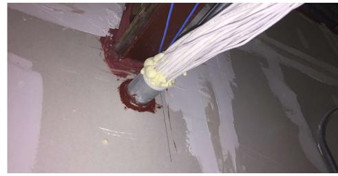
· A non-firestop foam has been used inside the conduits
