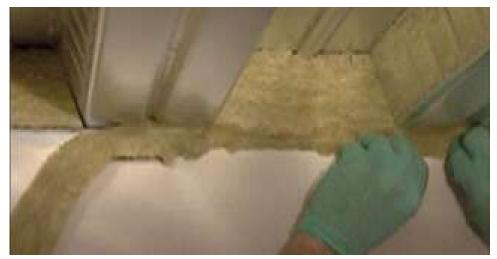
· Head of wall joints: Mineral wool grain should run horizontal
