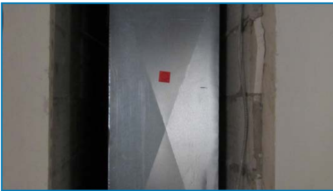
New shaft duct in a vacant shaft on the 4th floor.
