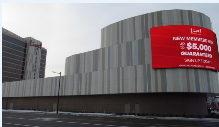
View from the corner of Packer Ave of the hotel with accommodations of more than 200 luxurious rooms and 30 suites.
