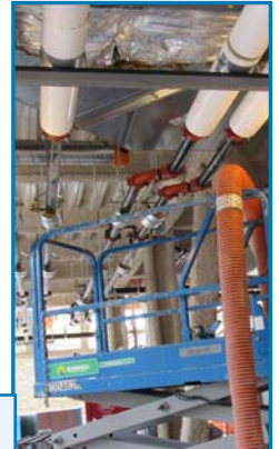
Leak Test first floor.
