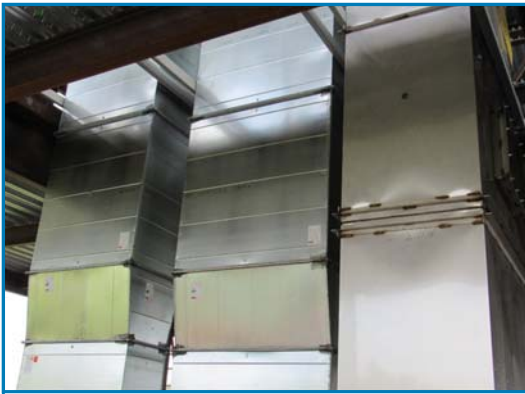
Here is one section of risers that were installed.
