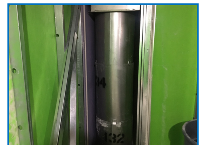
Trash shoot installed goes from the 8th – 47th floor.
