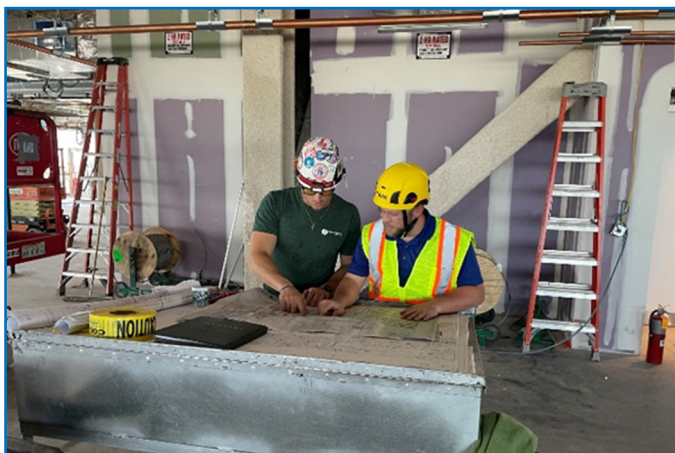
Foreman, Jeff Deckert and Project Manager/Sketcher Brad Kaighn review plans.
