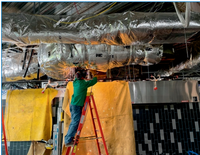
RVD President, Glen Armstrong, sealing ductwork.
