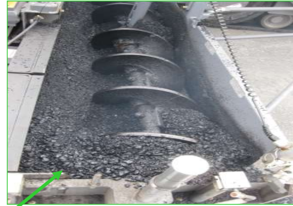
Running Augers too low
