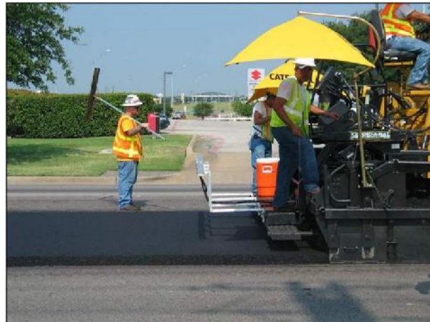
CORRECT SQUARE JOINT -- END GATE DOWN
