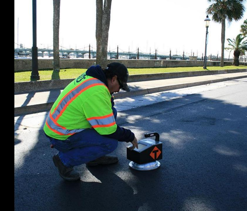
Check all joints and the mat for smoothness with manual or rolling straightedge
