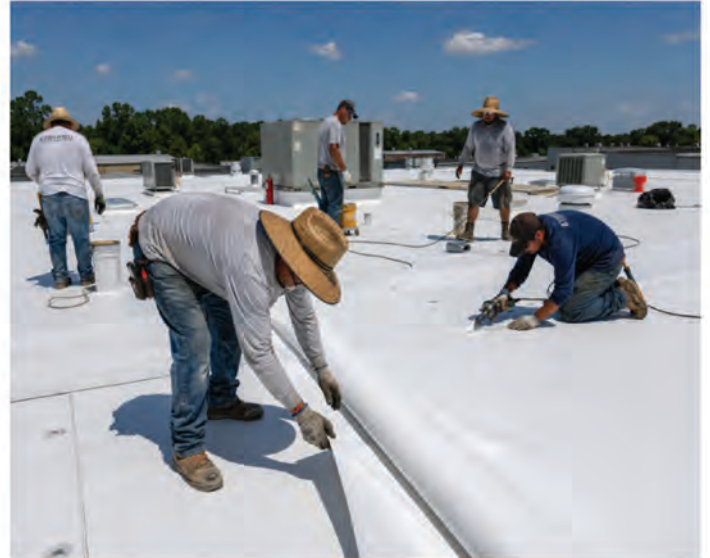
Lionheart Roofing crew at work on a commercial building rooftop.
