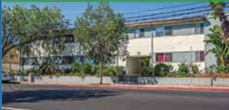
111 N La Cumbre Rd, Santa Barbara 17-unit apartment in Upper State area
