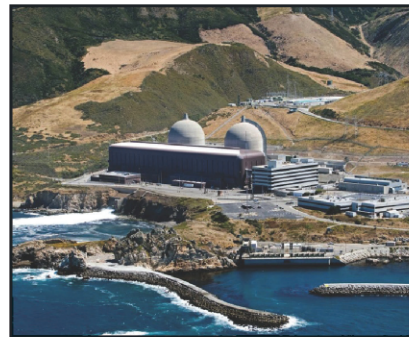
Diablo Canyon Nuclear Power Plant, image LATimes.com
