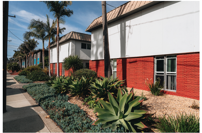
A Link-managed property at 6754-6764 Abrego Rd in Isla Vista
