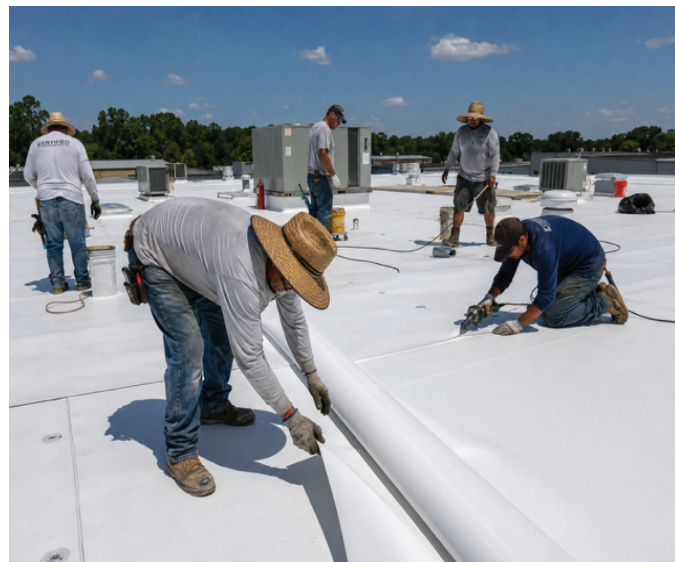
Lionheart Roofing crew at work on a commercial building rooftop.
