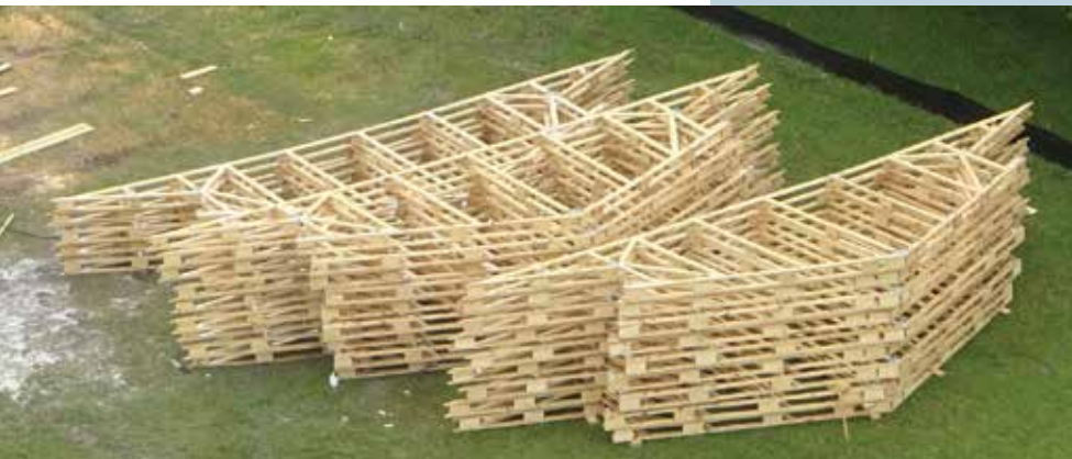
Figure 4. At the jobsite, the components were assembled into box beam trusses that consisted of a two-ply truss with 2x6 segments nailed in between the truss.
