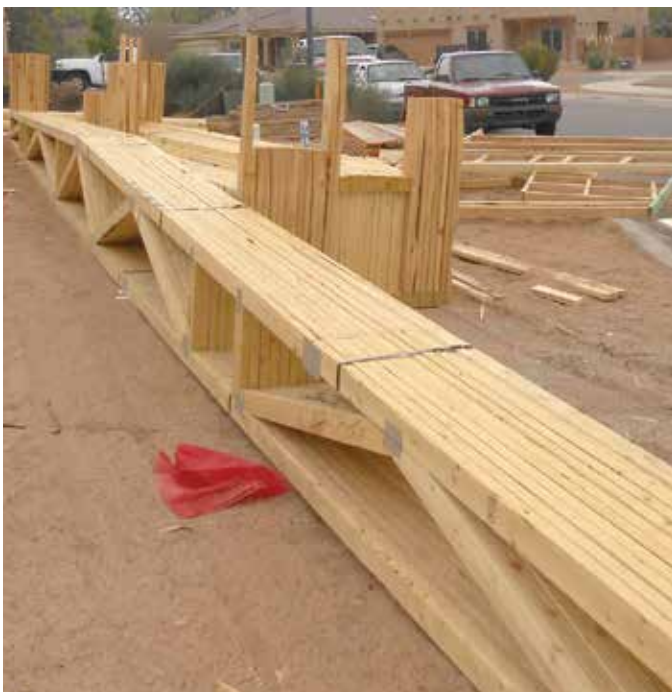
Figure 4. Parapets can either be manufactured into the truss design (as shown above), or they can be manufactured as stand-alone pieces.
