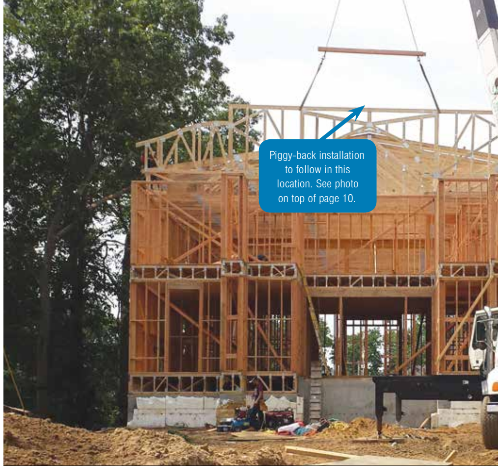
Figure 3. Installation of the roof trusses at the Spruce Street Shul. The curved peak of the building was manufactured in two segments that were piggybacked at the jobsite.
