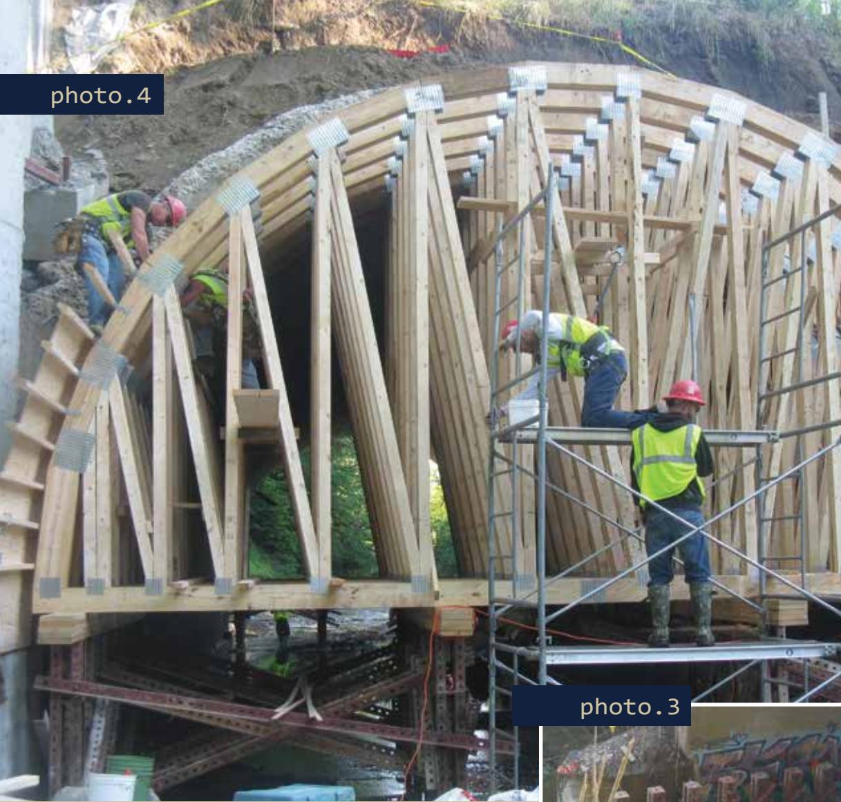
3. A platform of steel jacks were an integral part of the installation 4 & 5. The jacks provided four bearing locations for the truss assembly along their 28-foot length.
