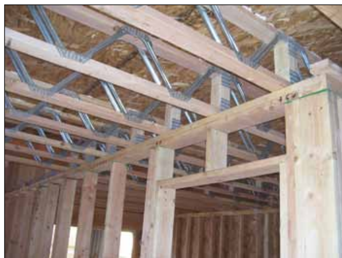
Photo 3. Open metal-web joists were used for the floor.
