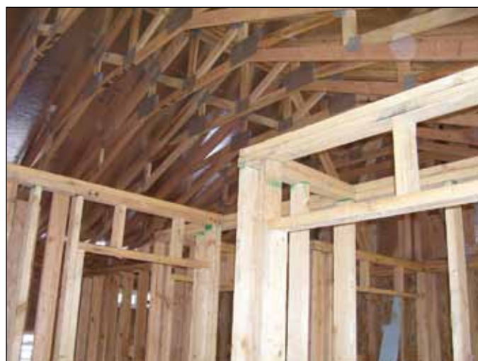
Photo 2. Scissors trusses were used to hang the mechanicals.
