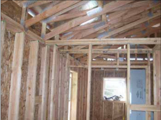
Photos 4 and 5. Examples of the result of using LSL to evenly distribute the load over the top plate. Note the lack of headers above doors and windows.
