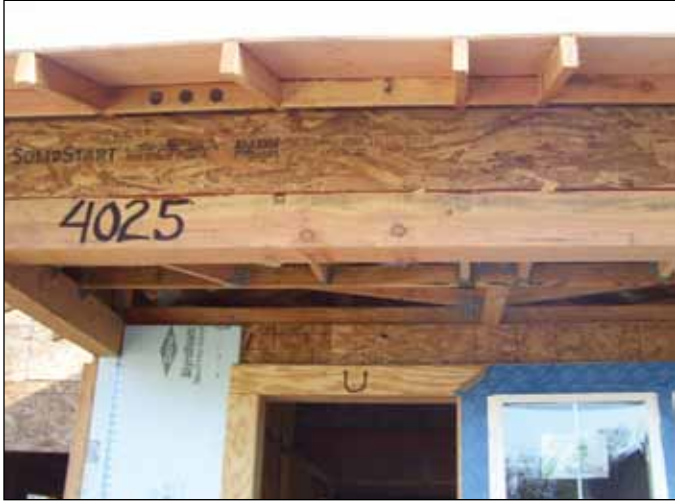
Photos 4 and 5. Examples of the result of using LSL to evenly distribute the load over the top plate. Note the lack of headers above doors and windows.
