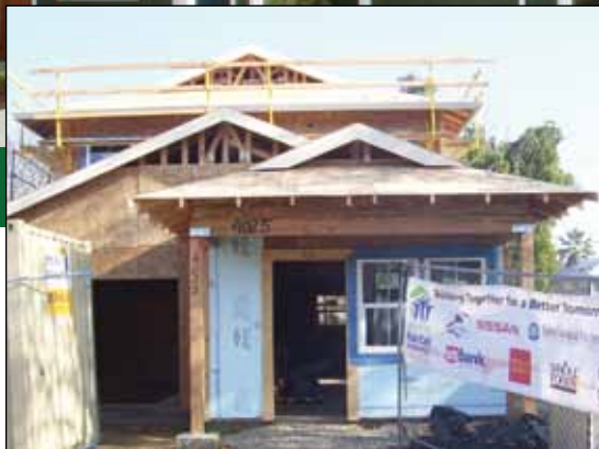
Photo 1. Habitat for Humanity Sacramento's net-zero house under construction. The blue house pictured above represents how the home will look upon completion.
