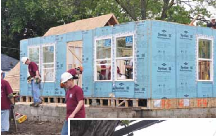
Photo 3. First floor walls were installed on the floor deck.
