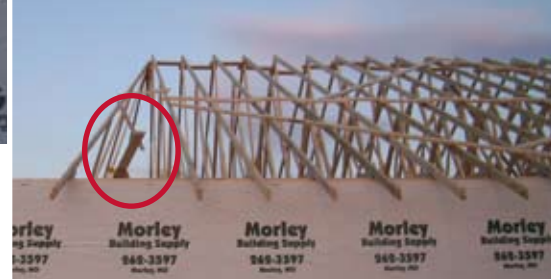
Top chord lateral restraint is visible in the photos above.
